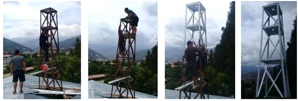
(A) (B) (C) (D) Once the tower was erected, additional elements (metal plates) where welded (A) to aid in installation of mast which holds the antenna rotator and the antennas itself. The tower was then painted (B & C) to prevent corrosion and rusting. The picture (D) shows the tower after completion of the aforementioned works.
