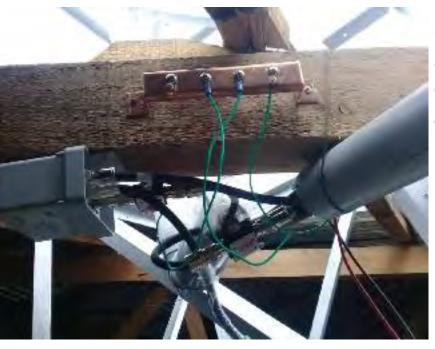
(*Right*) The Power cable for the amplifier is modified to meet the power supply arrangement.
