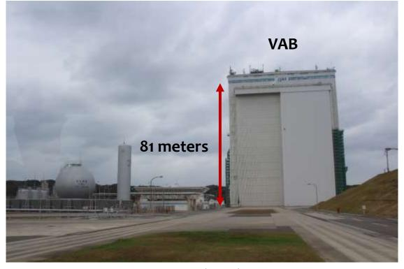
**Vehicle Assembly Building (VAB)** is a facility to assemble, outfitting, and inspect a launch vehicle shipped from a factory. At the VAB, two vehicles can be assembled simultaneously. The launch vehicles are assembled on a large-scale launch vehicle movable launcher (ML). The satellite and fairing are mounted, and the vehicle is transported to the launch pad. Source: http://global.jaxa.jp/activity/pr/brochure/files/centerso2\_e.pdf
